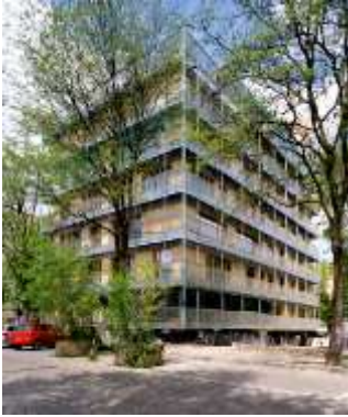
Photo 4: Building project R50 (Photo credits: Andrew Alberts)
